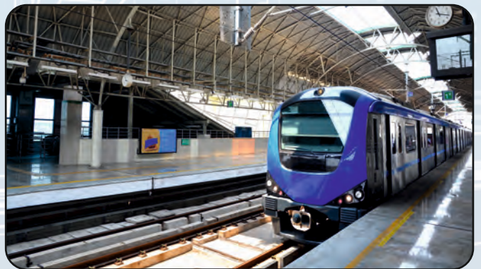
India: Chennai Metro Rail Project (UAA-01 & UAA-05) (Tunnel Length 5.7Km & 11.36Km) Scope: Detailed Design
