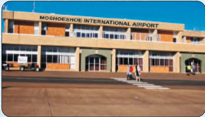
Lesotho: Moshoeshoe 1 International Airport Scope: Economic Feasibility, Detailed Engineering Design & Airport Master Planning
