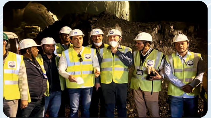
India: Zojila Tunnel (Length-13.145Km) Asia's longest Single Tube Bi-Directional Tunnel at an altitude of 11578 ft. above MSL Scope: Authority Engineer for Construction Supervision
