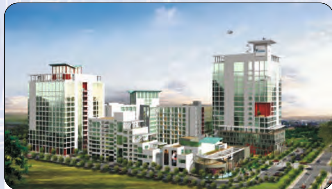
India: Information Technology Park at Manesar Scope: Construction Supervision & Project Management
