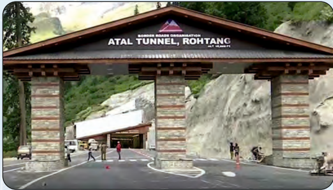
India: Atal (Rohtang) Tunnel, Length - 9.02Km World's longest Single Tube Bi-directional Tunnel at an altitude of 3000M above MSL Scope: Construction Supervision
