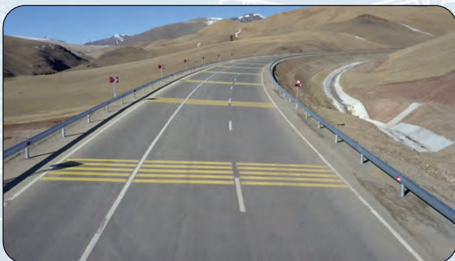
Mongolia: Western Regional Road Corridor Investment Program (2 Lane, 232.24Km), ADB funded Scope: Construction Supervision under FIDIC Conditions of Contract
