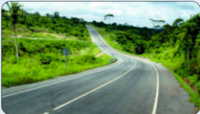
Ghana: Fufulso-Sawla Road Project (147.50Km), AfDB funded Scope: Construction Supervision
