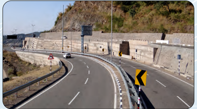
India: NH 22, Zirakpur-Parwanoo Section (4/6 Lane, 28.4Km) Scope: Independent Engineer/Construction Supervision
