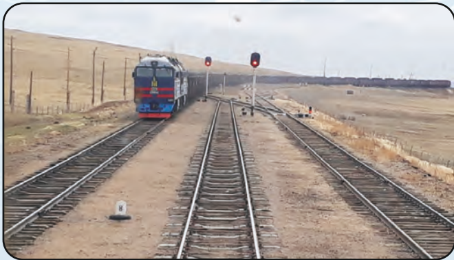
Mongolia: Bogdhan Railway Bypass Investment Program-01 (Length: 166.44Km, including 3 Tunnels of Length 15.16Km), ADB funded Scope: Alignment Study
