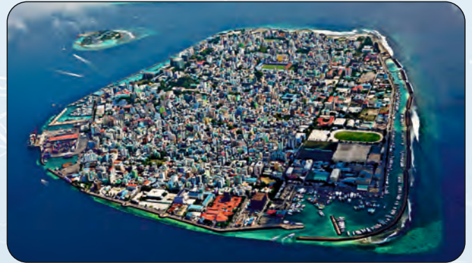
Maldives: Regional Development Project Phase II, ADB funded Scope: Environmental Infrastructure & Management
