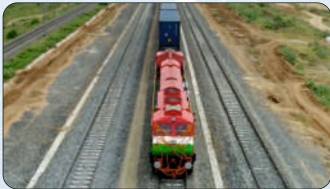
India: Eastern Dedicated Freight Corridor Project (Khurja-Dadri Section) (Length: 94.56Km), World Bank Funded Scope: Project Management Consultancy under FIDIC Conditions of Contract
