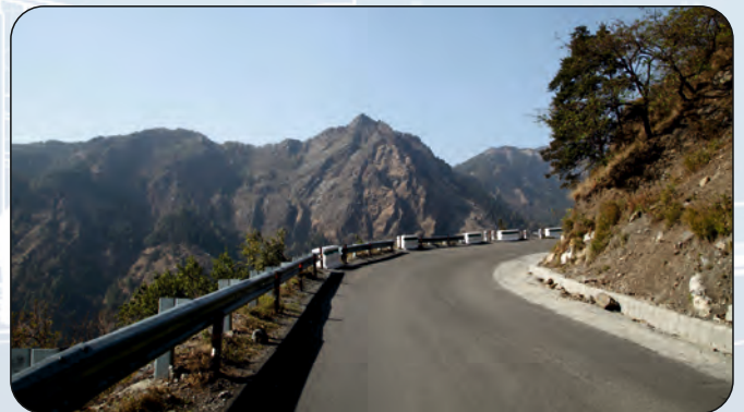
India: Himachal Pradesh Blackspot Improvement Program, World Bank funded Scope: Detailed Design & Bidding Documents for the Prioritized Engineering Interventions
