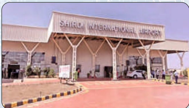
India: Shirdi Airport Scope: Project Management Consultancy
