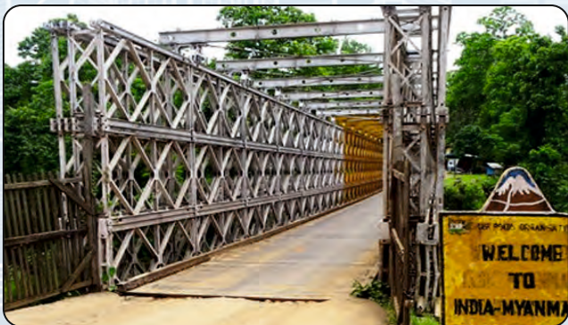
Myanmar: Tamu Kyigone Kalewa Road Section of Trilateral Highway Scope: Detailed Design of 69 Bridges
