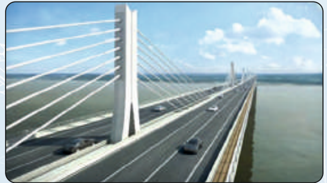
India: Phaphamau Bridge over River Ganga (6 lane, 3.839Km-Extradosed) Scope: Feasibility Study, Detailed Design & Construction Supervision
