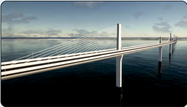
India-Extradosed PSC Bridge over River Brahmaputra, (4 Lane, 3.6Km) Scope: Project Management Consultancy
