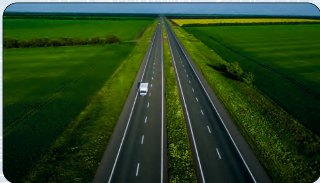
Vietnam: Ben Luc-Long Thanh Expressway (4 Lane, 58Km), ADB funded Scope: Design Review & Construction Supervision under FIDIC Conditions of Contract
