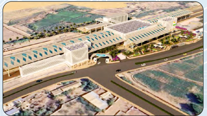
India: Bhuj and Rajkot Railway Station Scope: Authority Engineer for Construction Supervision
