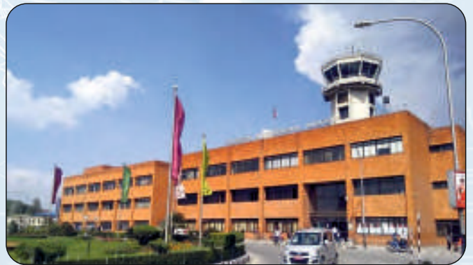
Nepal: Tribhuvan International Airport, Kathmandu, ADB funded Scope: Construction Supervision
