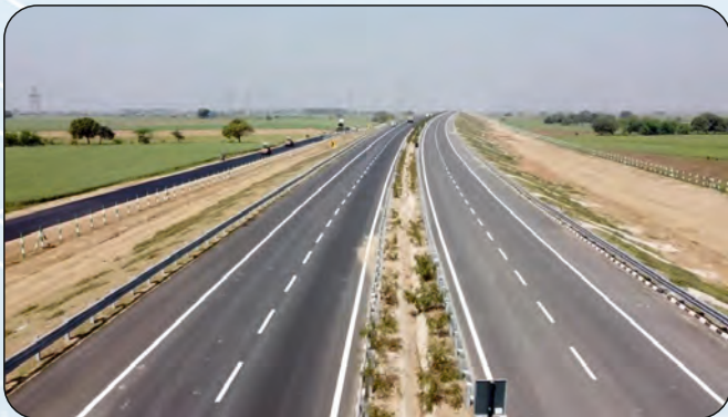
India: Bundelkhand Expressway (4/6 Lane, 296.06Km) Scope: Authority's Engineer for Construction Supervision
