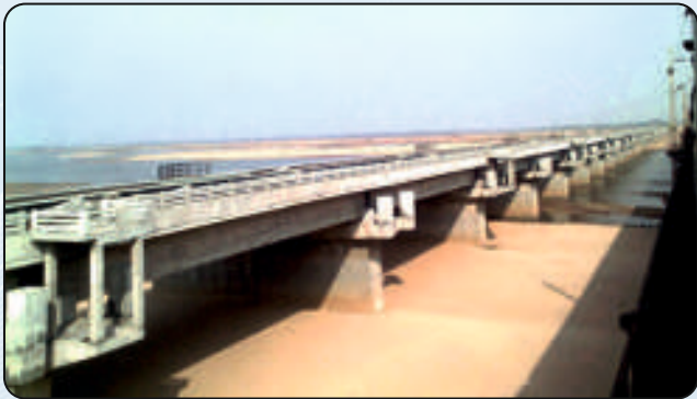
India: Sone Bridge (3.06Km) Scope: Project Management Consultancy
