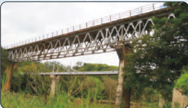
Tanzania: Wami Bridge, Length 513.50M Max. Span 120M Pier Height 58M Scope: Feasibility Study & Detailed Design
