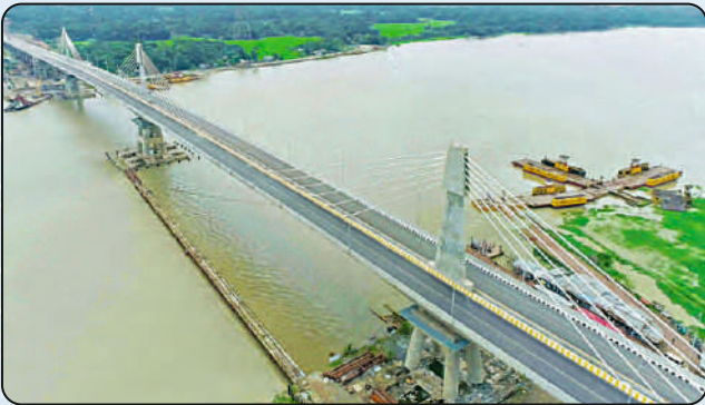
Bangladesh: Paira Bridge (4 Lane, 1.47Km - Extradosed), KFAED funded Scope: Detailed Design, Bid Management & Construction Supervision
