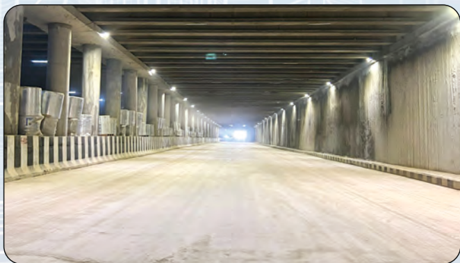
India: Dwarka Expressway (8 Lane Shallow cut and cover Tunnel, Length-3.6Km) Scope: Authority Engineer for Construction Supervision
