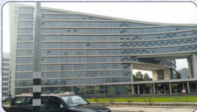
Bangladesh: Roads & Highways Department Headquarter 13 Storied Building, ADB funded Scope: Construction Supervision
