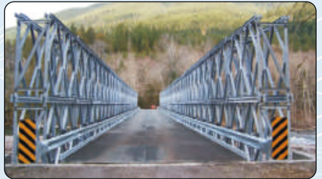
India: Uttarakhand Disaster Recovery Project, World Bank funded Scope: Detailed Design Introduced India's First Two Way Acrow Bridge of 60M
