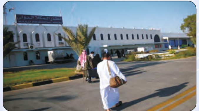
Yemen: Mukalla International Airport, World Bank Funded Scope: Construction Supervision of Terminal Building
