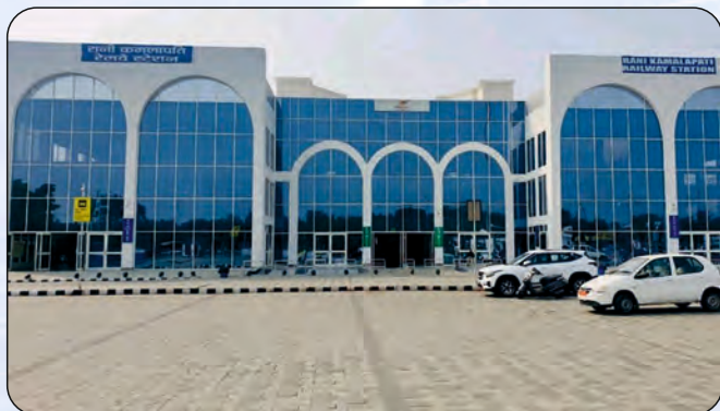
India: Rani Kamalapati Railway Station (Formerly known as Habibganj–Bhopal Railway Station) Country's First World-Class Railway Station Scope: Technical Feasibility Study & Master Plan
