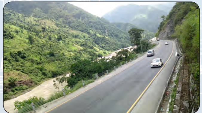
Nepal India Regional Trade and Transport Project, World Bank funded Scope: Road Safety Audit, Feasibility Study, Detailed Design including 2 Lane Single Tube Tunnel & Construction Supervision under FIDIC Conditions of Contract
