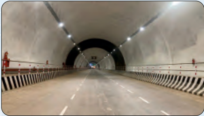
India: NH-47, Vadakkancherry-Thrissur Section (Twin Tube Tunnels, Total Length-1.925Km) Scope: Independent Engineer for Construction Supervision
