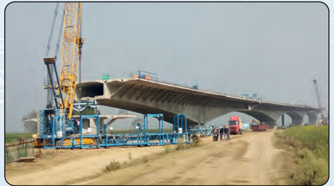
India: Bakhtiyarpur Bridge (4 Lane, 5.55Km) Scope: Independent Engineer for Construction Supervision
