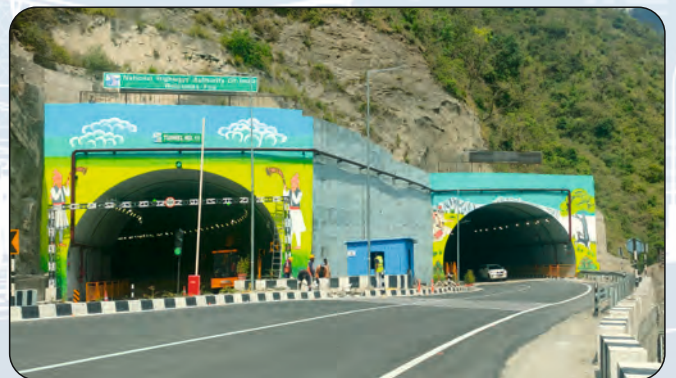
India: NH-21, Pandoh Bypass -Takoli Section (Single & Twin Tube Tunnels, Total Length-11.638Km) Scope: Independent Engineer/Construction Supervision
